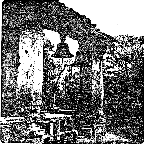
Plate XXIX. The bells of Cal Barrio church.
